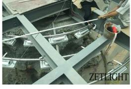
Left and below are pictures of a ZetLight installation at the Foshun Hilton Hotel in Guangdong (formerly Canton), China. This shows some of the lighting suspended on circular rails above the 9 metre x 5.5 metre high acrylic aquarium and the finished product, complete with walkway to a lounge on top of the aquarium – doesn't everyone have one of those?
